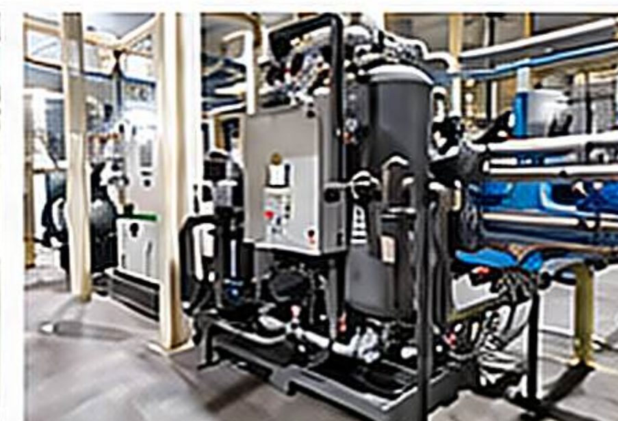
End User Food & Beverage Equipment Heatless dryer 4 sets (45 m³/min per set, 40 bar)
