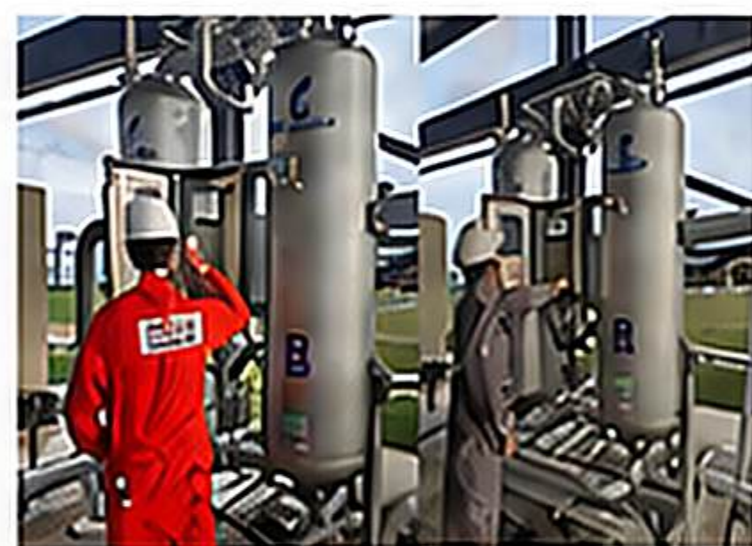
End User Chemical Plant Equipment Heatless dryer 1 set (40 m³/min)
